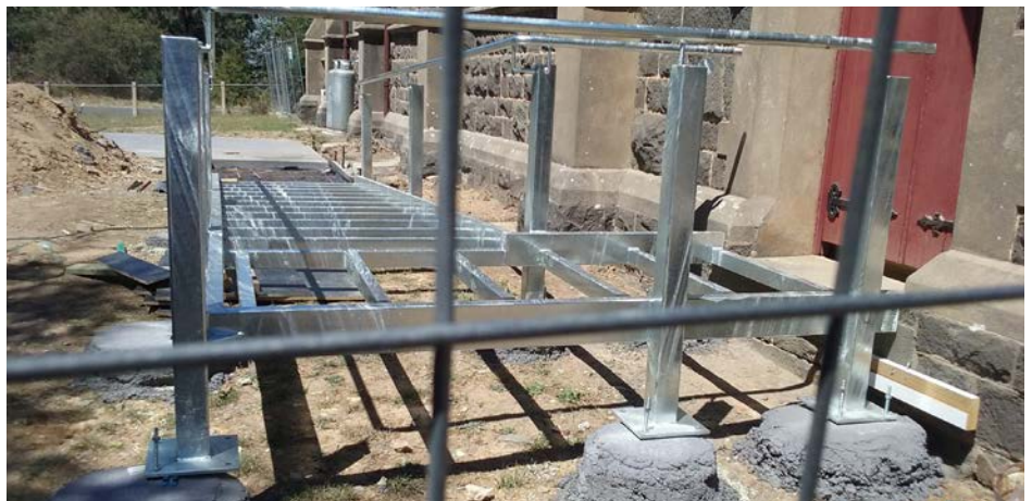
Under construction: The framework for the access ramp
